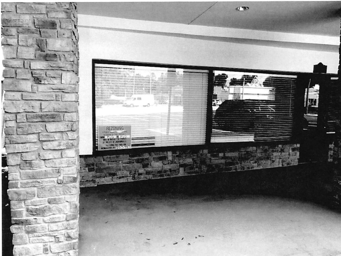
View of building
